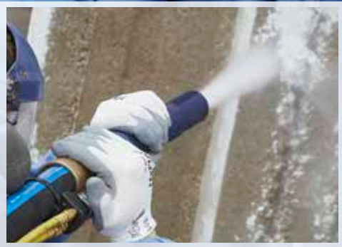
Concrete Surface Preparation
